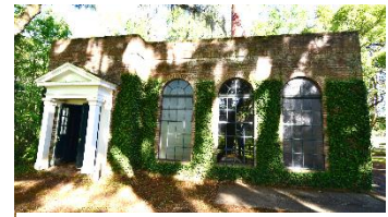
The Pump House building exhibits the concrete, steel, brick veneer technique common on the property.
