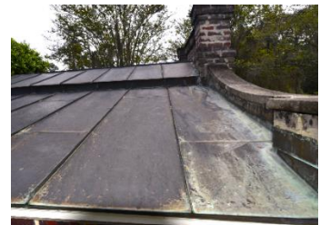
Diverse materials like the raised seam metal roofing on the Kitchen Garden Shed.
