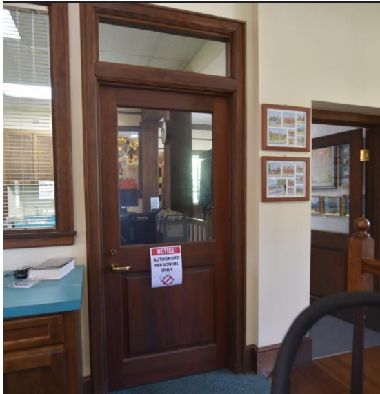
Fig.II.181 The modern doors are solid core with panels.
