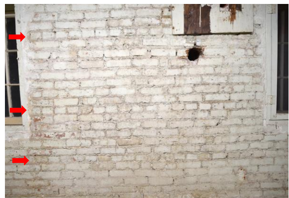
Fig.II.26 The American bond pattern rotates every 6th or 7th course (red arrows) perpendicular to the wall plane.
