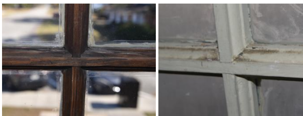
Fig.II.194 The muntins (1 st floor on left, basement on right) are slightly larger at the base than other Arts and Crafts style profiles.
