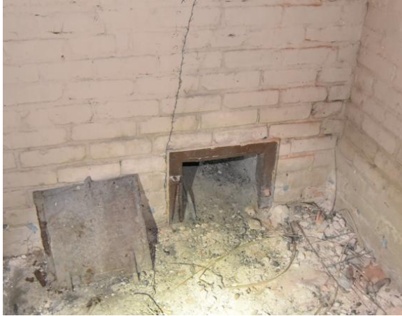
Fig.II.149 Ash trap in old exterior basement wall.
