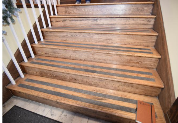
Fig.II. 230 Evidence suggests these stairs are not the building's original stairs.
