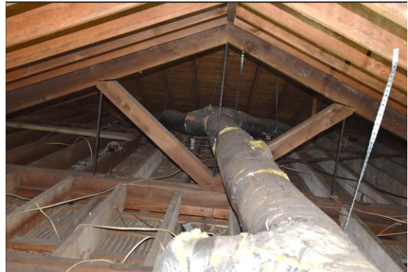
Fig.II.56 A single large timber roof truss is located approximately 19' from the south end of the building.
