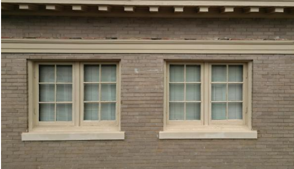
Fig.II.189 The side elevations have double sash configurations.
