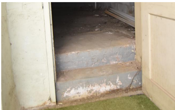
Fig.II.178 These stairs ascend to what was once the original height of the exterior grade. Today, it is well below the existing grade height.
