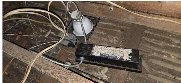
Fig.II. 244 High intensity discharge fixtures light the main reading areas.
