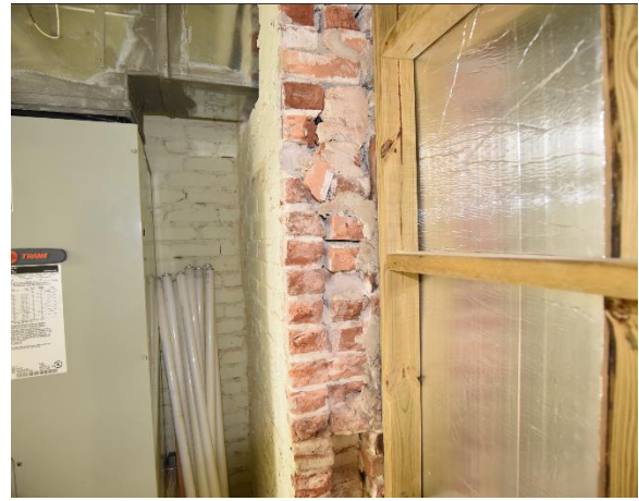
Fig.II.25 Inner load bearing walls in the historic structure are two wythes of common red brick run in a American bond pattern.
