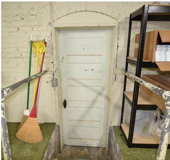
Fig.II.173 Door to northside storage room is original Note the arched opening in masonry wall..
