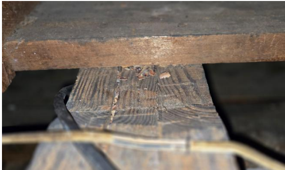
Fig.II.64 Many of the ceiling joists have hand cut notches to accommodate the rafter plate.
