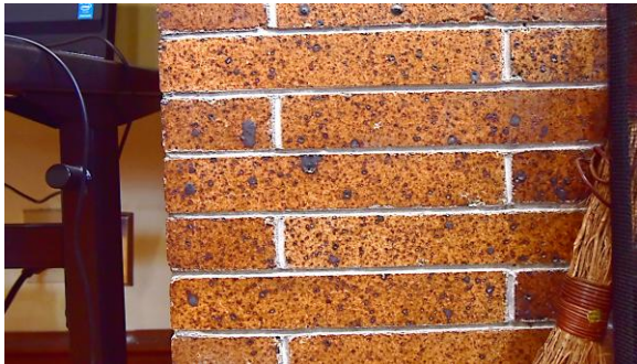
Fig.II. 150 "Ironspot" bricks were used for all visible surfaces.
