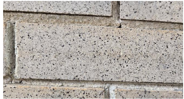
Fig.II.21 The black specks may be manganese added during manufacturing.
