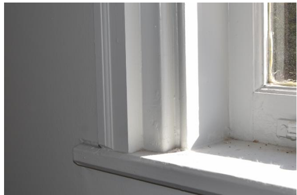
Fig.II.200 Windows in southside function room have a combination of historic elements and modern components. The trim on these windows was "built out" to accommodate the wall board added during renovation.
