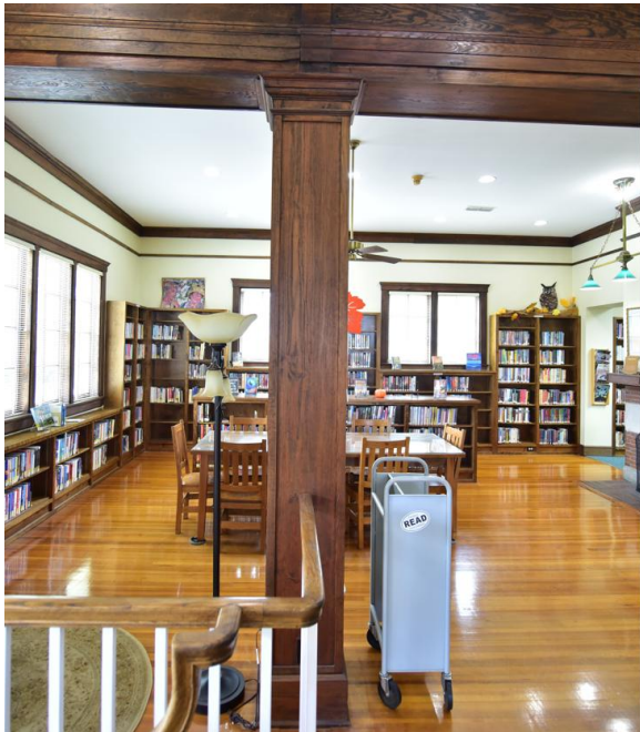
Fig.II.137 Pillars are topped with a crown molding detail and a skirt at the bottom.
