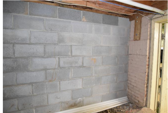
Fig.II. 28 Modern addition walls are CMU laid in running bond pattern.
