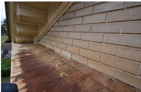
Fig.II.69 A small roof section within the pediment covers the lower section of the entablature.
