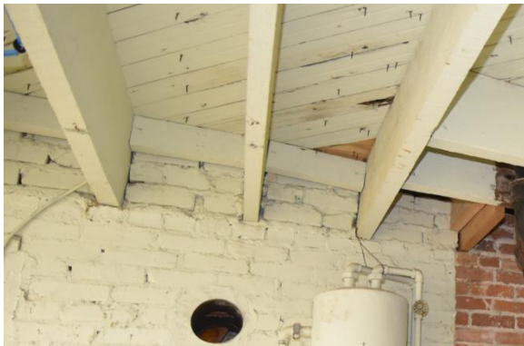
Fig.II.47 Floor joists sit in masonry pockets along the perimeter.
