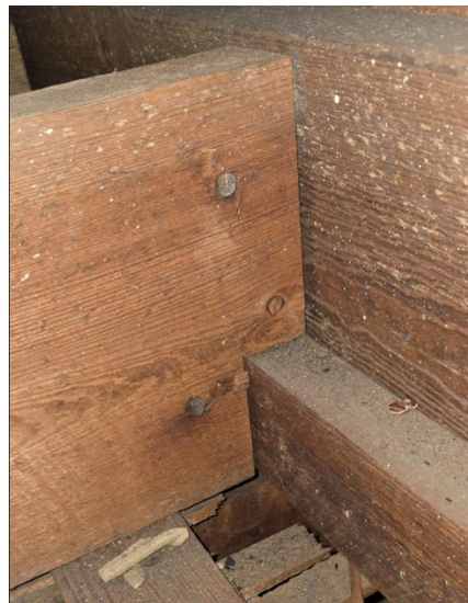
Fig.II.49 Ceiling construction on south side likely mirrors floor framing system below. Joists are notched over a ledger board fastened to carrying beam.
