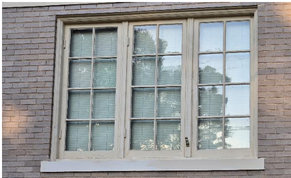
Fig.II.186 The historic windows are a character defining feature of the building.
