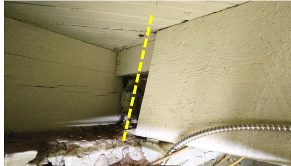
Fig.II.48 Floor joist exhibit an angular "fire cut" at end of timber. This was a common safety measure in the age of widespread structure fires.
