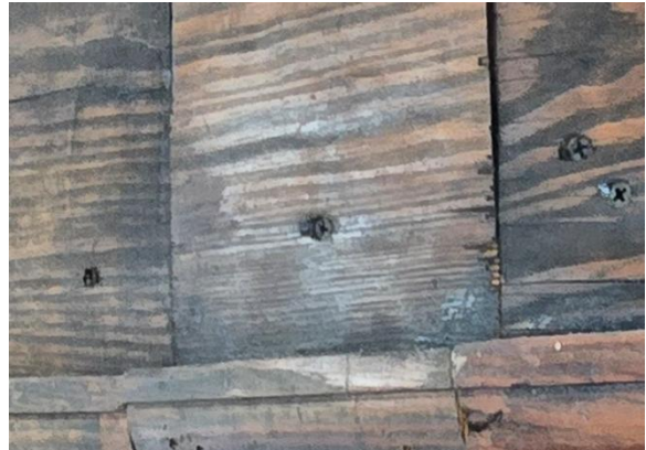
Fig.II.155 Repairs to the beams were fastened with drywall screw in a hasty arrangement.
