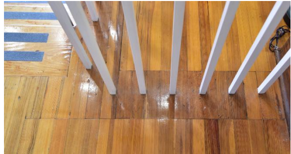
Sec. I/ Fig. 55 Discoloration of flooring shows original wall location.
