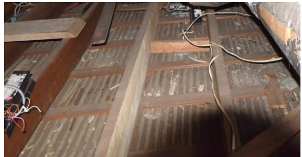
Fig.II.160 Attic view of back side of original plaster and lath ceiling.
