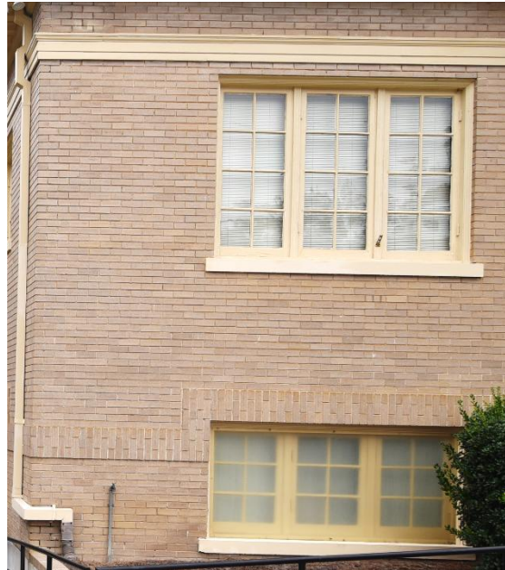
Fig.II.9 Exterior walls are single wythe of buff colored brick laid in a running bond pattern.
