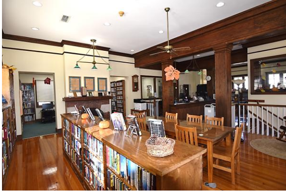
Fig.II.132 The beams and pillars in the public space are decorative, not structural.
