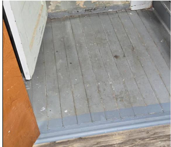
Fig.II.223 The floor at the bottom of the basement stairs is historic.
