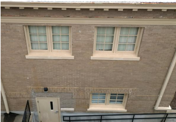
Fig.II.190 The basement openings are smaller and one was converted to a doorway.
