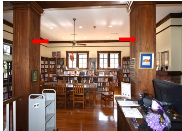
Fig.II.61 Long tie rods enclosed in decorative columns on first floor.
