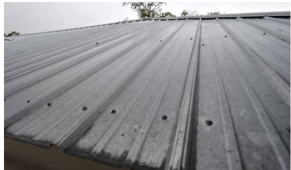
Fig.II. 67 36" ribbed metal panels are the roof finish.
