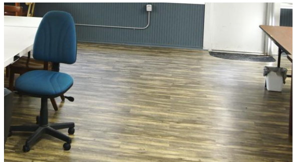
Fig.II. 224 The southside rooms have a vinyl plank covering installed sometime after 2015.
