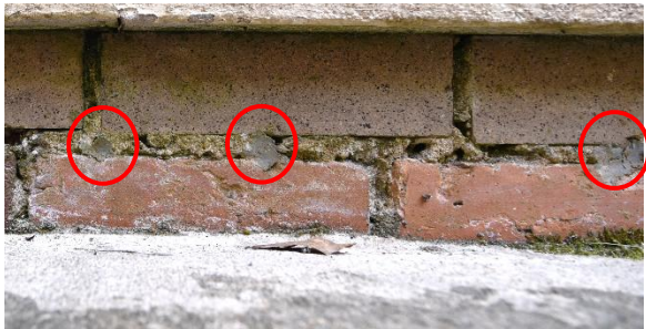
Fig.II.35 Weep holes in historic exterior walls patched.
