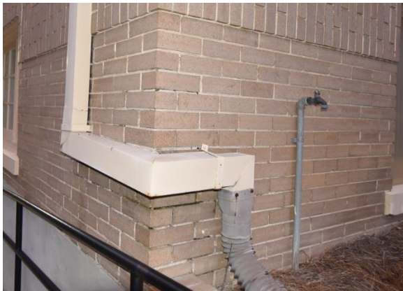
Fig.II.87 Front downspouts have been re-routed to direct water into ground on east elevation.
