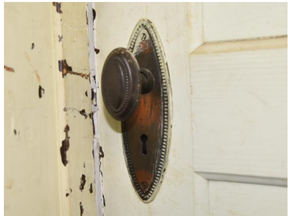
Fig.II.175 Original hardware in good working condition but some overpaint.
