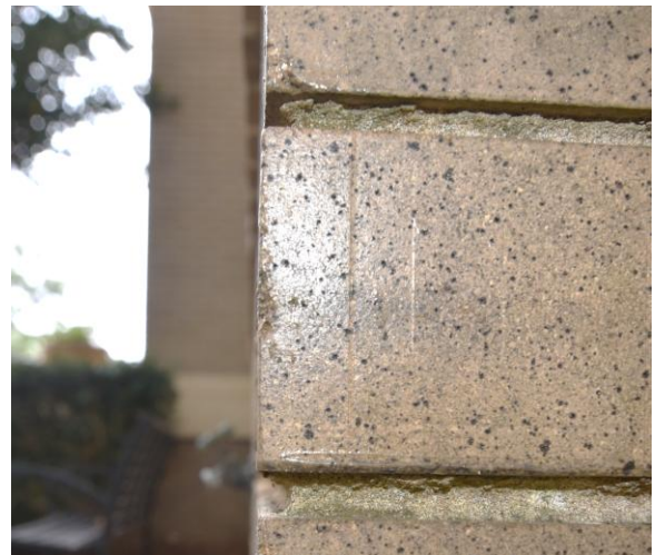
Fig.II.22 Mortar exhibit both Vee and raked profiles.
