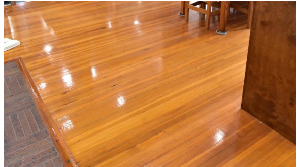
Fig.II.213 Flooring is a tongue and groove with a 2 1/2" face.
