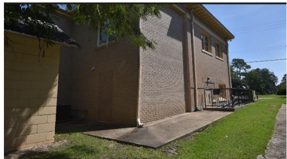
Sec. I/Fig. 46 Concrete walkway/apron wraps around southwest corner of building.
