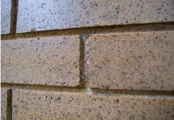
Fig.II.19 Face bricks reflect their box formed, early 20th c. manufacture.
