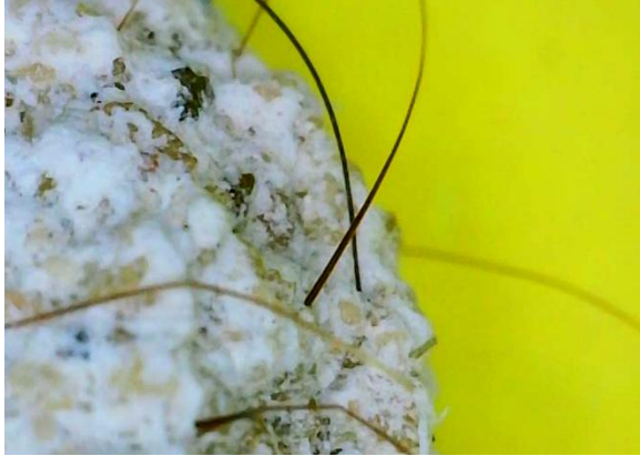
Fig.II.102 Horsehair was used as a binder in the plaster throughout the building. A basement sample under 10x magnification.
