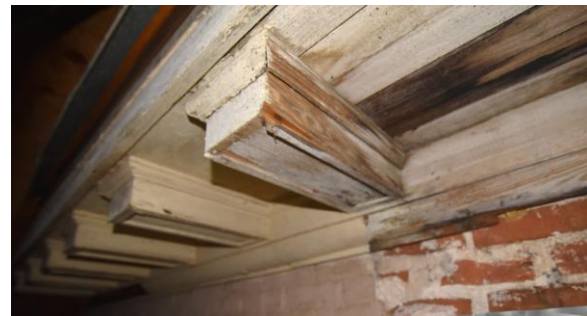
Fig.II.14 Original cornice on west wall was encased above the acoustic ceiling by 1993 Addition.
