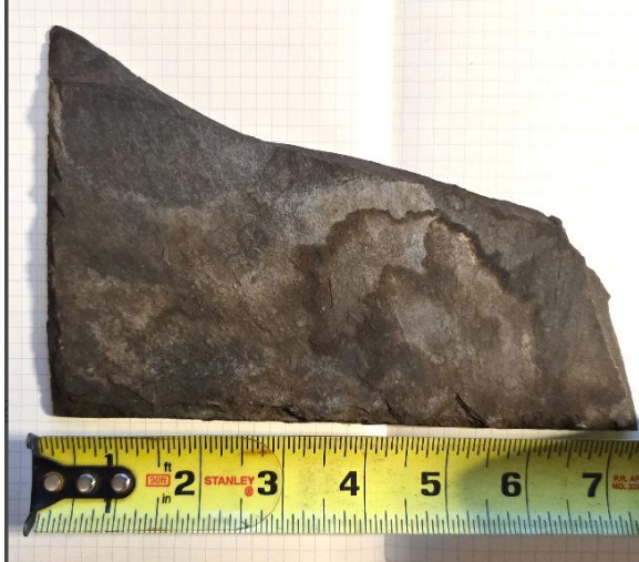
Fig.II.74 Portion of an old slate roof shingle found in the attic below debris.
