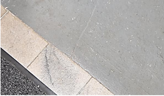
Fig.II. 220 The lack of visible wear on this heavily travel doorway (to basement) indicates materials are relatively new.
