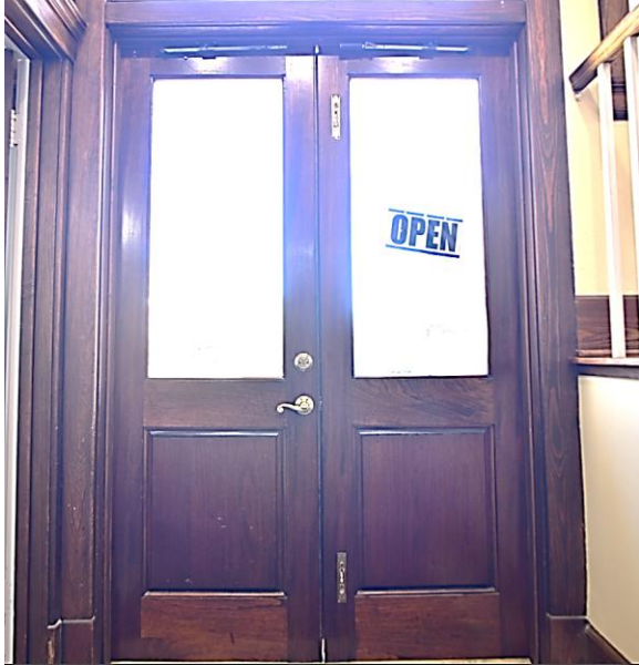
Fig.II.165 Doors are solid wood construction with a raised lower panel and a glass upper.
