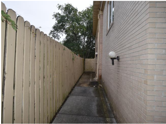
Sec. I/Fig. 43 Northside walkway looking east, toward Main Street.
