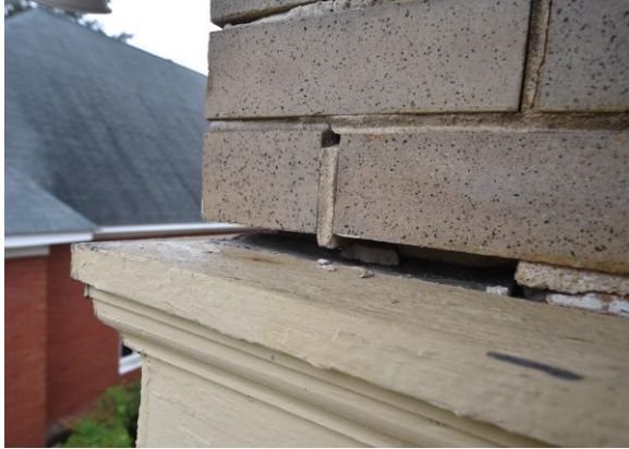
Fig.II.37 Above architrave in southeast corner.
