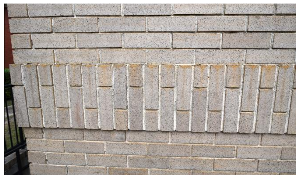
Fig.II.10 The lower horizontal belt element is a 12" Water table composed of vertically arranged stretcher bricks.
