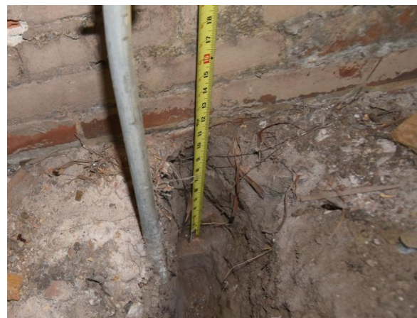
Fig.II.3 The building's spread footer is at varying depths below grade. At rear, footer is 12" deep.
