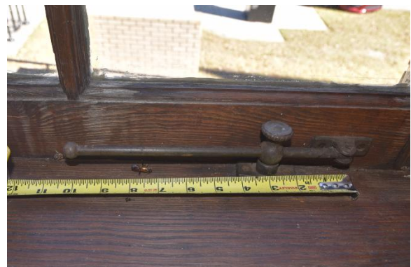
Fig.II.196 Much of the original hardware is intact and operational.
