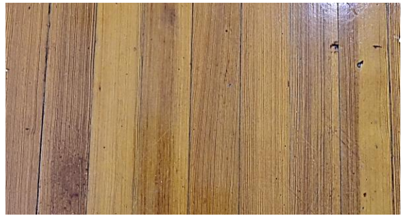
Fig.II.214 Floor uses quarter or rift sawn boards. Note the orientation of the grain.
