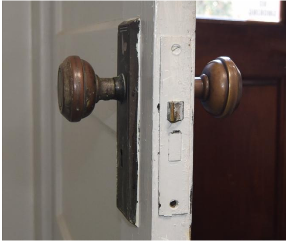
Fig.II.172 The historic mortised box lock is still well seated and secure.
