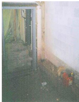
Sec. I/ Fig. 59 Construction photograph from 1993 Addition indicates floor was dug up, perhaps for plumbing, then raised to match doorway height.
