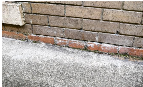
Fig.II.33 Another example of how red common bricks were used on exterior below grade or in non-visible areas.
