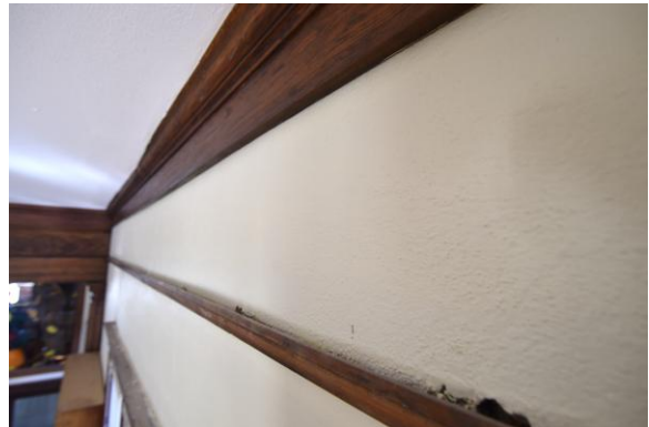
Fig.II.101 Plaster applied directly on brick, rather than wood lath, was used on all the historic perimeter walls and is still almost entirely intact.
