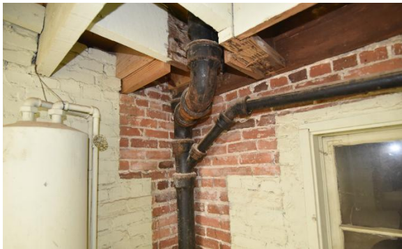
Sec. I/ Fig. 31 The original plumbing stack below the building's first bathroom survives in the basement.
