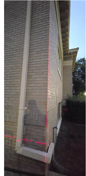
Fig.II.36 Laser tests indicate exterior walls are still relatively level and plumb.
