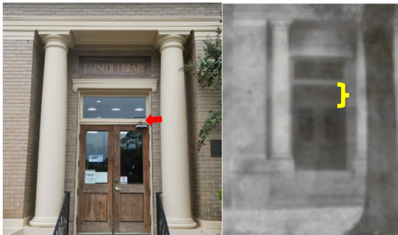
Fig.II.166 There is a significant dimensional difference above the glass panel in the historic photo versus the same
