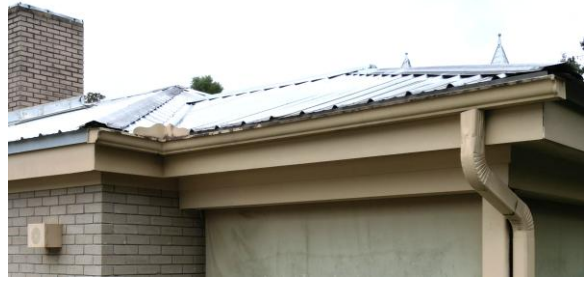
Fig.II.88 K gutters and downspouts serve much of the modern addition roofing.
