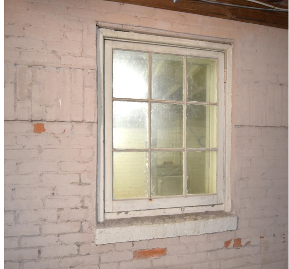
Fig.II.191 One of the historic 9 light windows in the basement.
