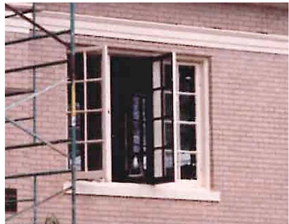
Fig.II.188 An undated photograph (ca early 2000s) shows these casement windows in an open position.
