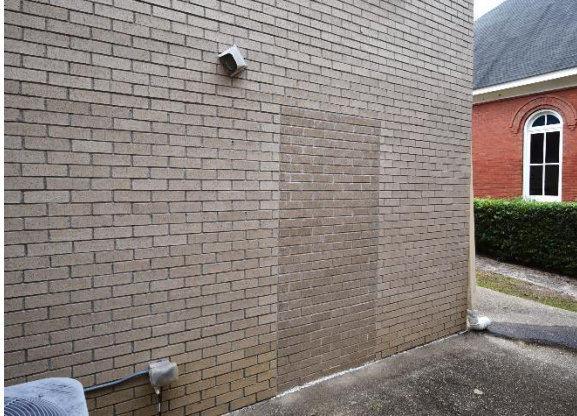
Fig.II. 34 In-fill of basement doorway on west elevation. Exact date unknown.
