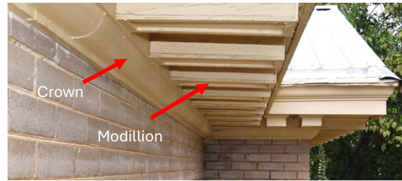
Fig.II.13 Modillions and crown molding detail the underside of the cornice.
