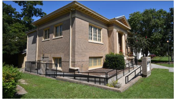
Sec. I/Fig. 45 ADA ramp and doorway added to southside of building.
