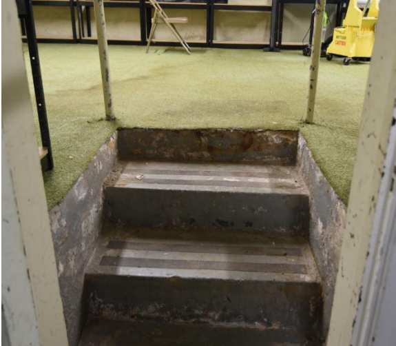
Fig.II. 225 The thickness of the raised concrete floor on the northside basement could not be determined.
