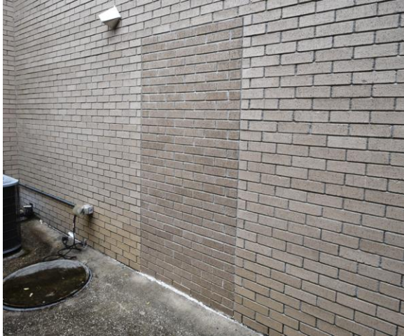
Sec. I/ Fig. 61 The 1993 rear exit was in-filled during the ADA ramp addition.
