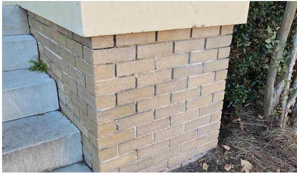
Fig.II.38 Southeast corner of northern cheek wall at entry
