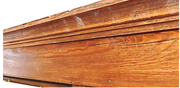
Fig.II.142 Top of door and window casings have a solid molding.
