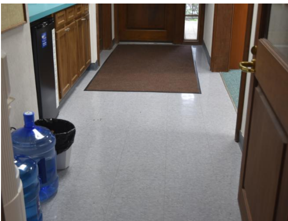
Fig.II.222 The hallway/kitchenette and restrooms have 12" vinyl tiles.
