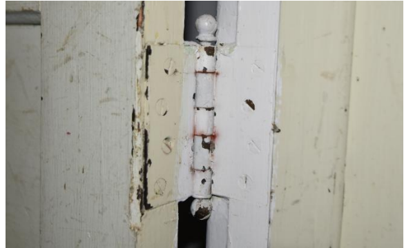
Fig.II.174 Door has original hinge mounting and assembly.
