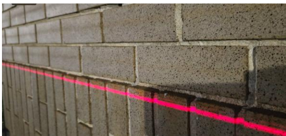
Fig.II.8 Laser suggests building is still remarkably level.
