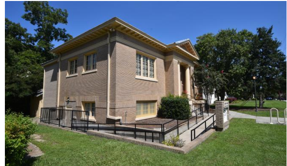
Fig.II.187 The proportion and balance of the windows give the overall building much of its historic character.
