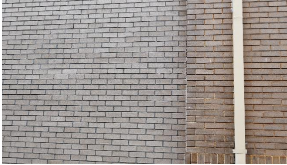
Fig.II. 23 Exterior bricks on Addition are nicely matched face bricks with a Portland cement mortar joint.
