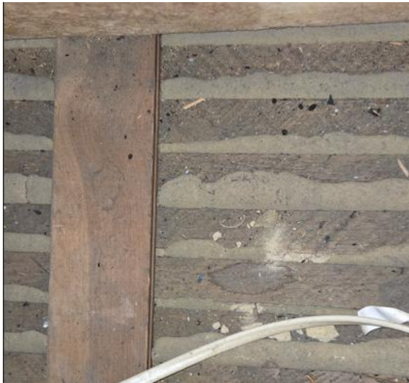
Fig.II.120 The ceiling on the other side of the building, over the south side reading area, was finished in plaster and lath the back of which is still visible.
