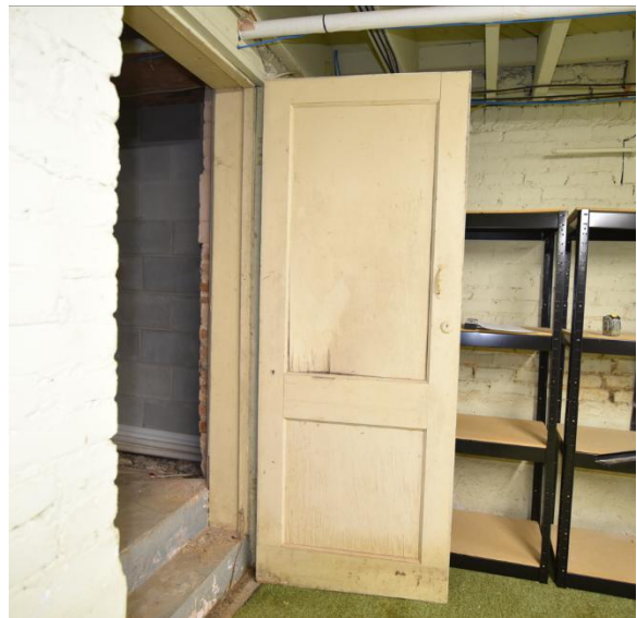
Fig.II.176 This was the building's original basement exit.
