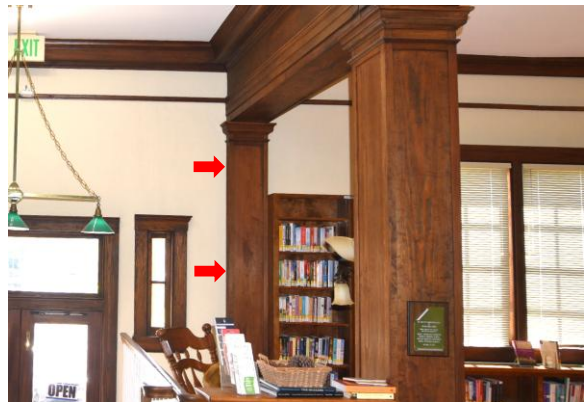
Fig.II.139 Half pillars (red arrows) originally finished the beam at the exterior wall plane. Only one of these survives.
