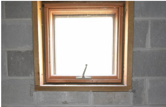
Fig.II.203 Window units in rear of Addition basement are awnings.
