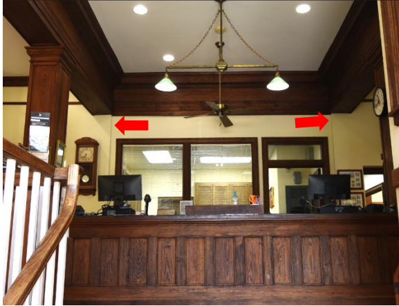
Sec. I/ Fig. 57 Outline of original "stacks" area still visible below the beams.
