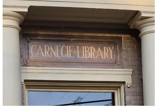
Fig.II.17 Limestone elements like the lentil above door are combined with terra cotta name panel.
