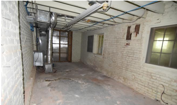
Fig.II.130 Original basement area below former "stacks" room.
