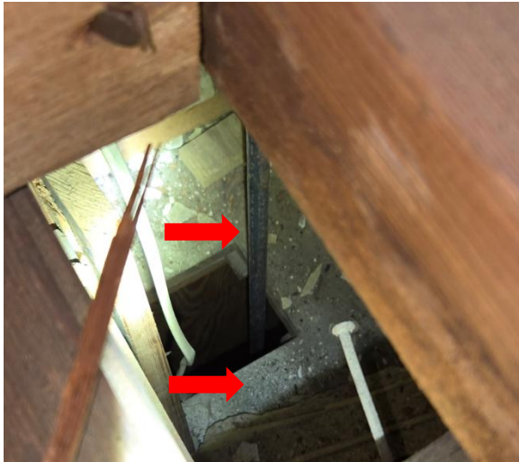
Fig.II. 59 One of the long tie rods (red arrows) that reach to the floor framing system 12' below.
