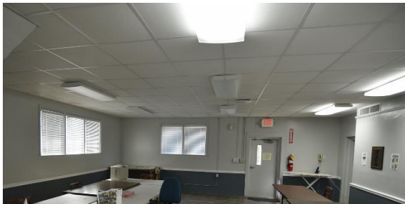
Fig.II.162 The acoustic ceiling in basement function room obscures the original plaster finish which is still intact.
