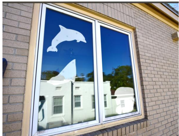
Fig.II.201 All the modern windows are vinyl-clad, double glazed, single light configurations.
