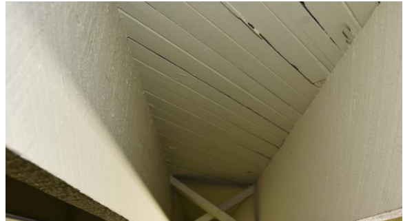
Fig.II.52 T&G subfloor still well fastened to joists.
