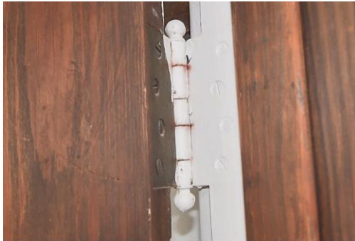
Fig.II. 169 Basement door jamb shows no evidence of prior mountings.
