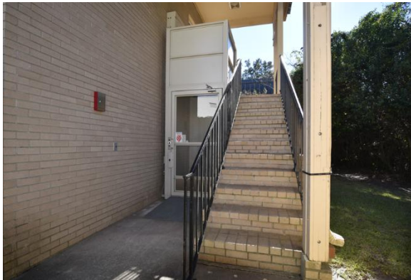
Fig.II.229 The rear stairway and lift were added sometime after 1993, likely as part of the ADA ramp project.
