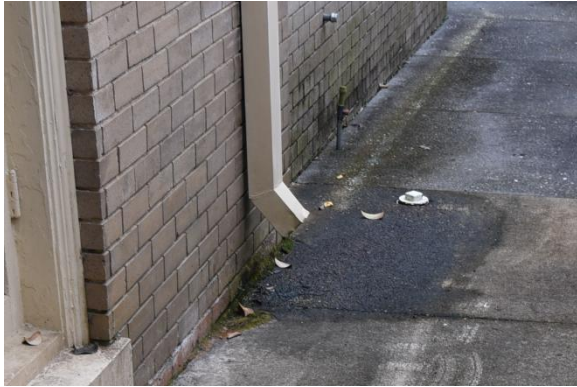
Fig.II. 86 Rear downspouts have elbow termination just above the apron.
