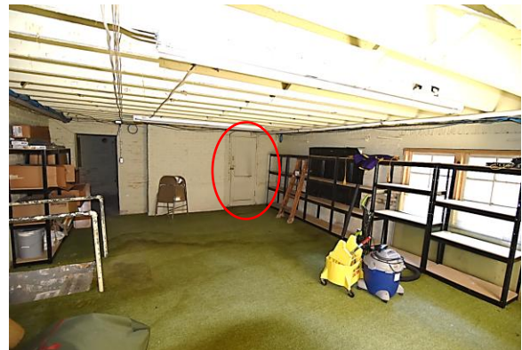
Fig.II.127 Northside basement is still a storage space, but original exit door (red circle) no longer serves as egress.
