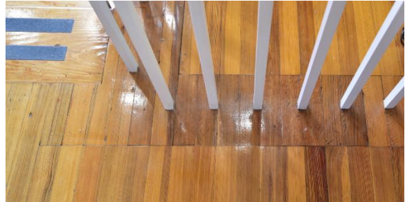
Fig.II.218 Patching where entry stairway wall once stood.
