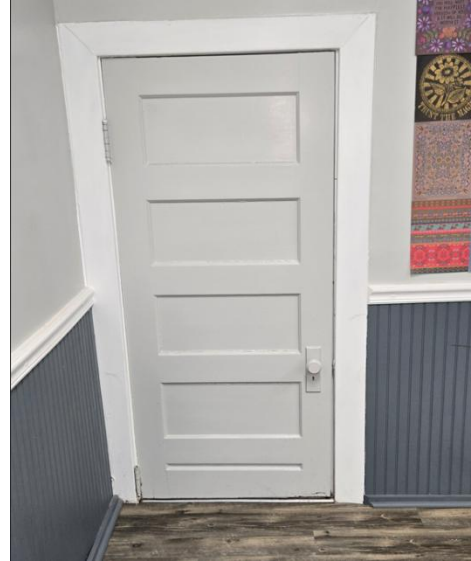
Sec. I/ Fig. 58 Narrow width of bottom door rail strongly suggests floor height was raised during the remodeling.
