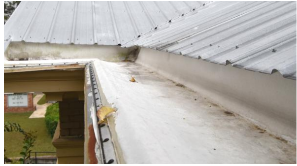
Fig.II.83 The box gutter has been modified with EPDM lining.
