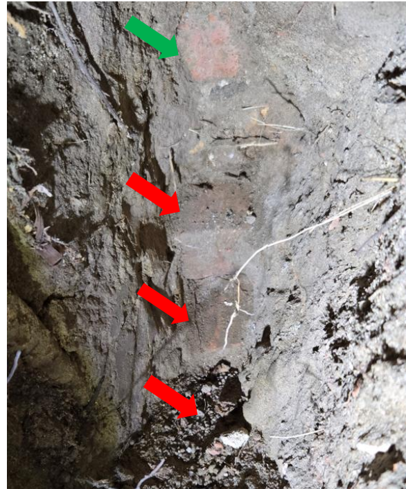
Fig.II.2 Excavation shows spread footer has three foundational courses below wall plane (green arrow).
