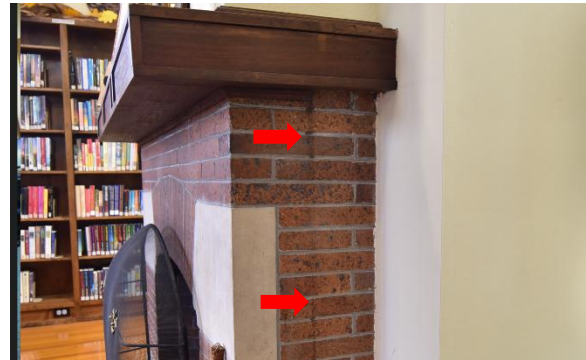
Sec. I/ Fig. 29 Ghost lines of wall bookshelves (red arrows) along chimney side.
