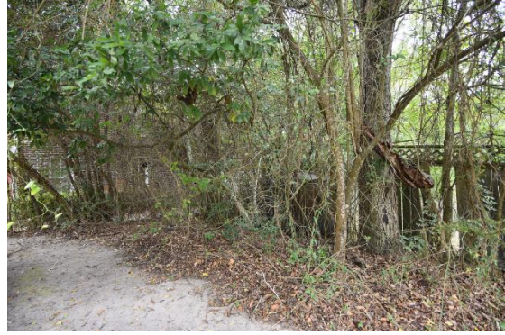
Sec. I/ Fig. 48 Extreme southwest corner of property is overgrown and bordered by deteriorated fence line.
