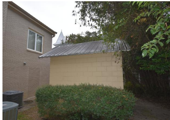
Sec. I/ Fig. 49 CMU storage structure in rear of library. Not evaluated for this report.
