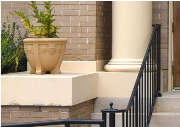
Fig.II.16 Limestone is used for the wall caps and columns as well as the base and capital elements.
