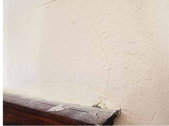
Fig.II.107 The plaster on brick walls, on the first story, are in excellent condition with only minor cracks observed.
