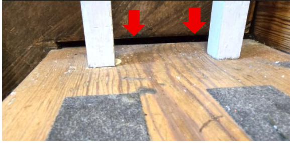
Fig.II.232 The gap (red arrows) between the skirt and the tread is not consistent with the workmanship exhibited in other historic elements.
