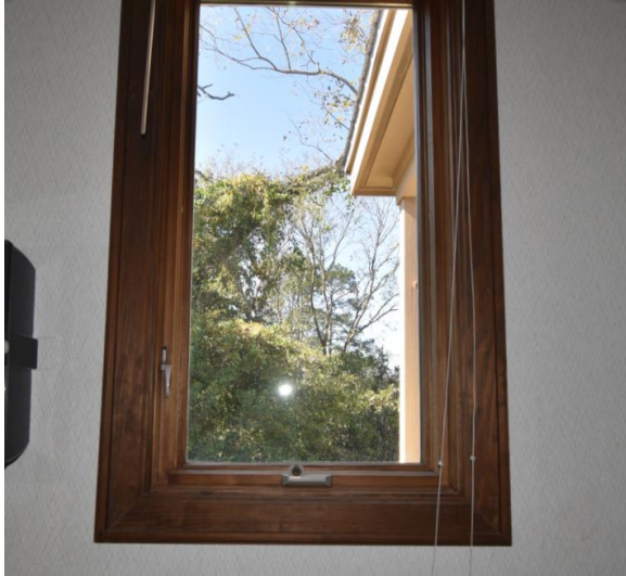
Fig.II.202 All but two modern windows are casements with hand crank hardware.
