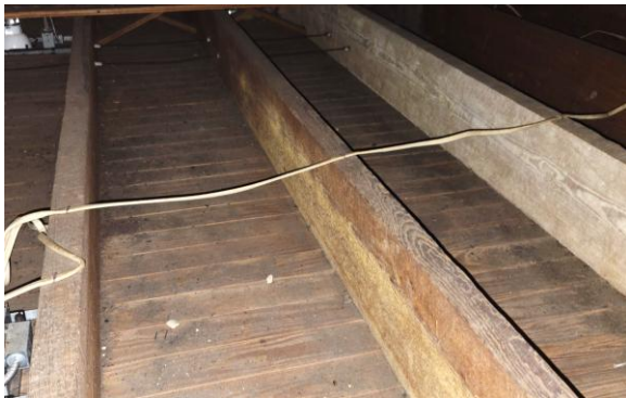
Fig.II.119 The original ceiling above the children's area was tongue and groove wood planking, the back of this material is still clearly visible in the attic.
