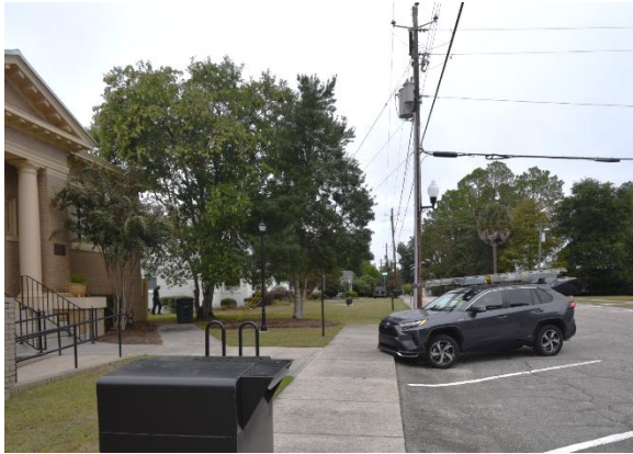
Fig.II.237 Electrical service for the building comes from a utility pole along S. Main Street. The line travels underground through a conduit to the northeast corner of the building.
