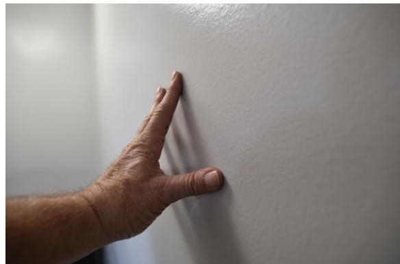
Fig.II.105 Multiple interior walls in the building are finished with gypsum (aka drywall) which has been taped, sanded and painted.
