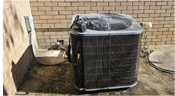
Fig.II.255 Compressor for 5-ton system.
