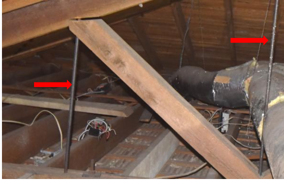
Fig.II.58 Two of the three threaded tie rods compressing the truss.
