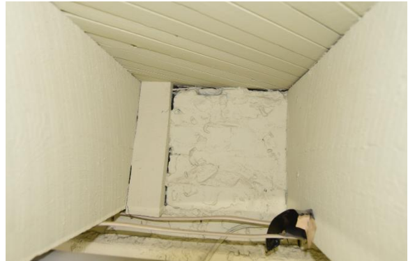
Fig.II.53 Joist pockets have good integrity.
