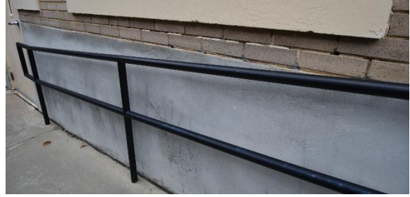
Fig.II.32 Lower portion of wall covered with skim coat of concrete.
